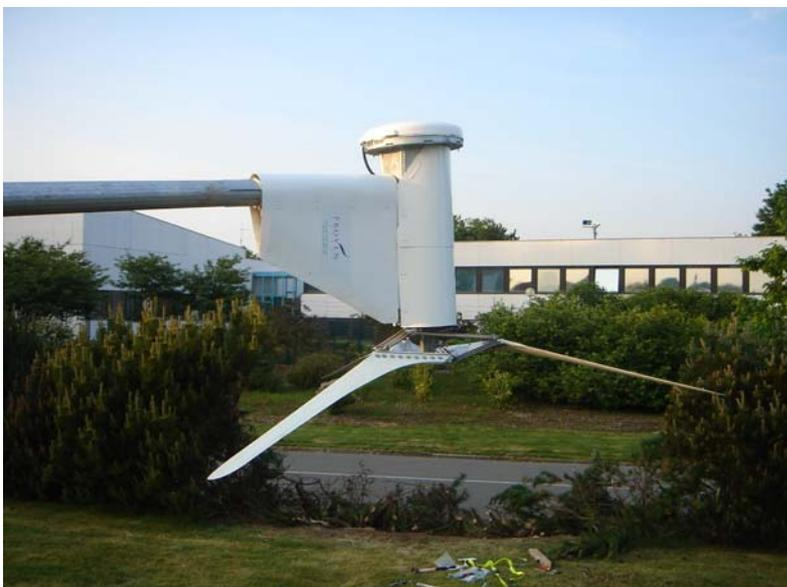
*Another couple of hours have gone by and the 3 blades are fitted, despite 3 seized nuts, an issue that is solved with proper tooling and the presence of spare parts in all Proven kits. Everybody on the site has gone home and the turbine is now ready to be lifted into upright position.*
